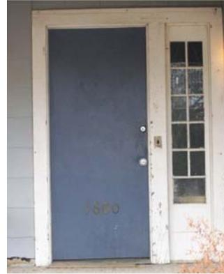
*LEFT, RIGHT AND BELOW: The transoms and sidelights of these examples have all been significantly altered by either being covered or removed. In some cases the original door has been removed and the opening has been reduced in size and the trim has been altered.*
