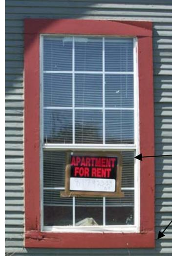
*Don't change the size of the original opening, surface mount the window unit or mitered the corners. It is inappropriate to change the size of the original opening. Traditional wood windows are recessed within the wall to allow space for shutters and screens. Mitered corners allow for water to seep behind the weatherboards, causing water damage to the wall.*
